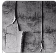
/ Wallpaper cracking
