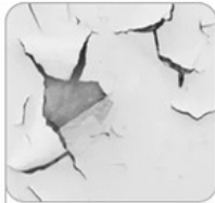
/ Cracking of the wall stucco layer
