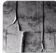
/ Wallpaper cracking
