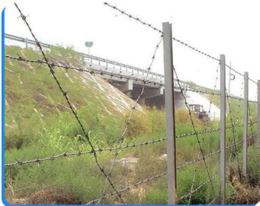
1. Attach the barbed wire on the concrete/wooden post with binding wire or nails.
