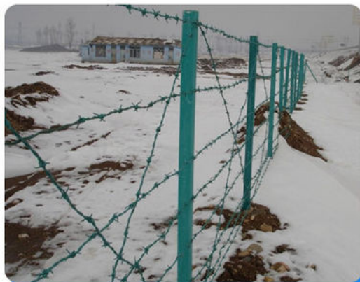
2. Hang the barbed wire on the hook, use a spanner to tension the span.
