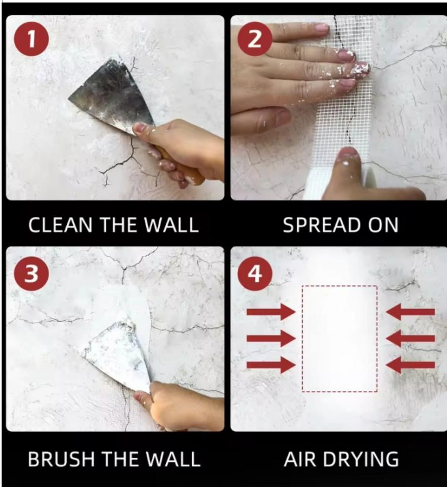
1. 75g / m2 mesh fabric used in the reinforcement of thin slurry, to eliminate small cracks and scattered throughout the surface pressure.
