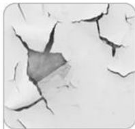
/ Cracking of the wall stucco layer
