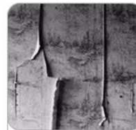
/ Wallpaper cracking
